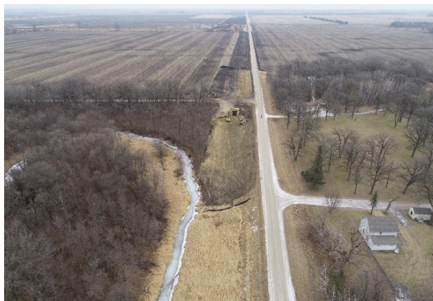
Outlet Channel Looking East (before)
