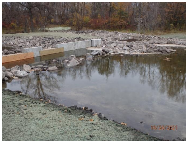
Outlet Structure without steel gates and catwalk
