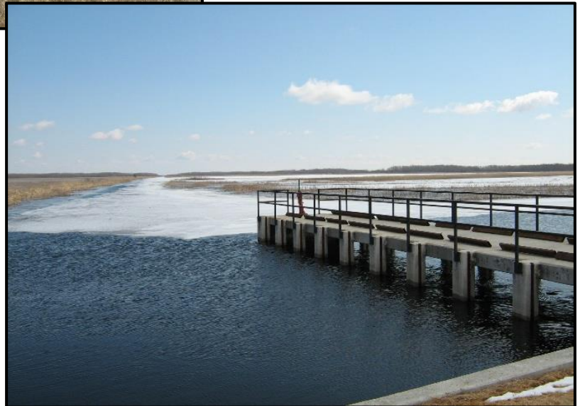
Example of an Impoundment with a permanent pool
