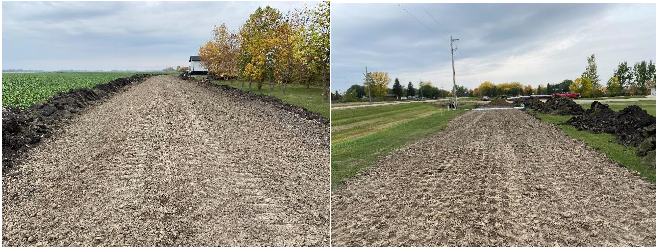
Looking east along north end of yard (during)
