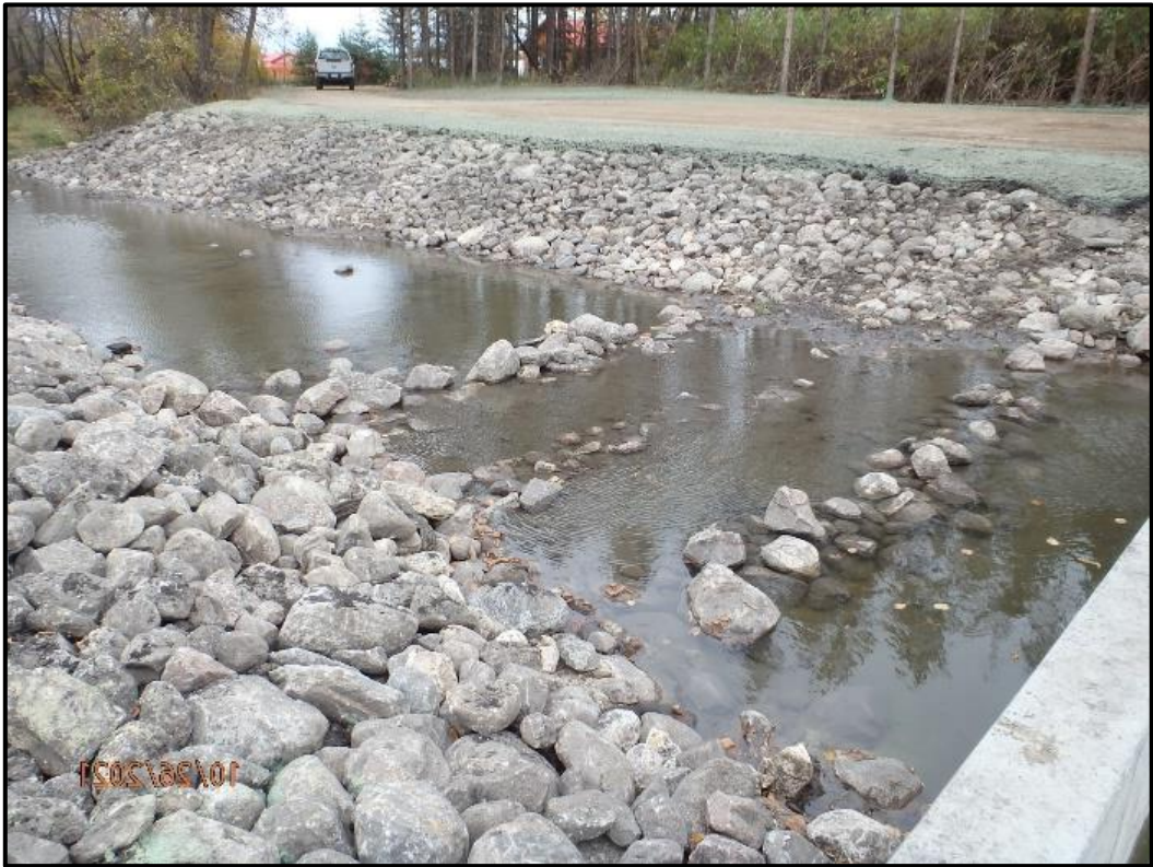
Riprap riffles downstream of concrete
