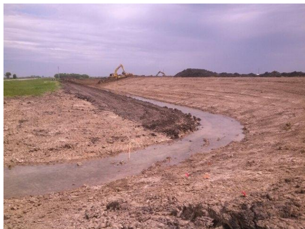
Ditch along TH #220 looking south
