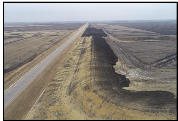
Looking East along south side CSAH #3
