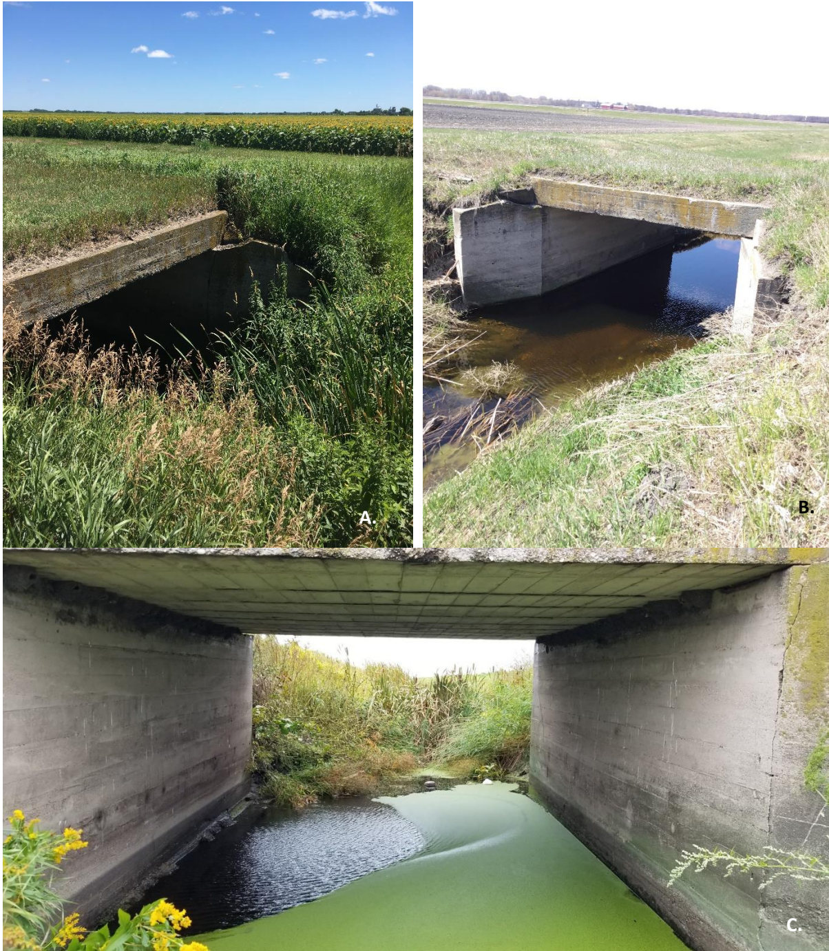
A. South west corner of failing bridge. B. East side of failing bridge. C. Under failing bridge, looking west.
