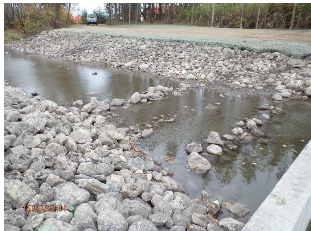
Fish Passage Structures
