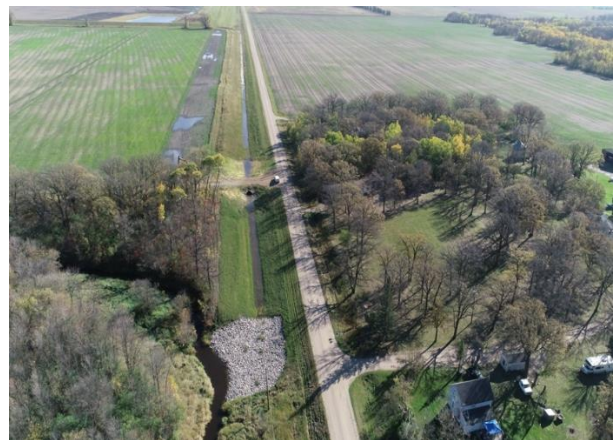
Outlet Channel Looking East (after)
