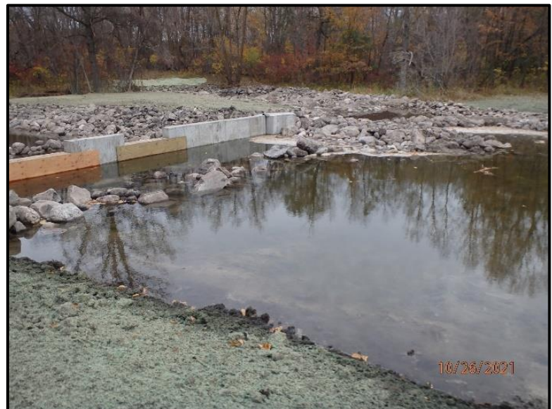
New structure without gates and catwalk.
