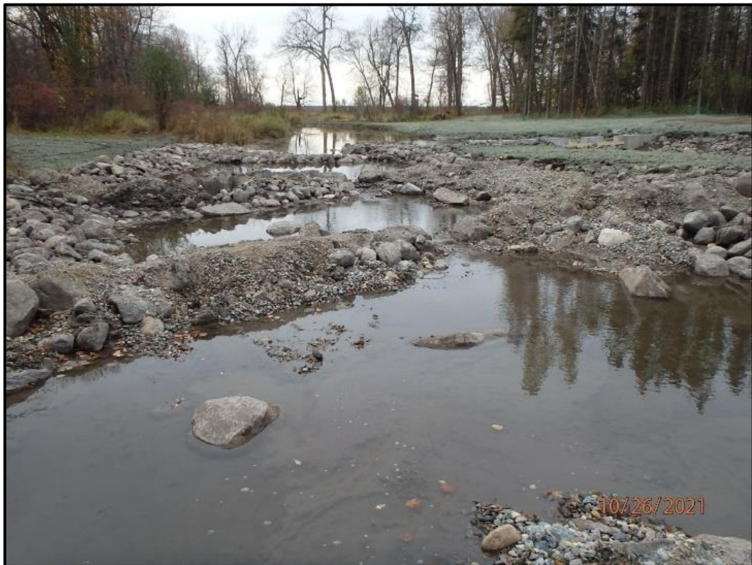
Looking up-stream at fish passage.
