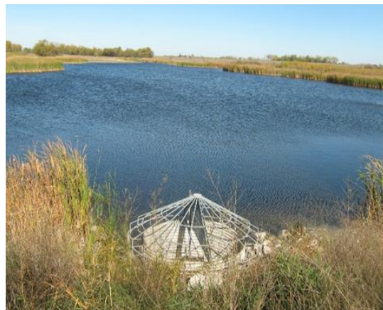
Odney Flaas Dam located in Onstad Township, Polk County
